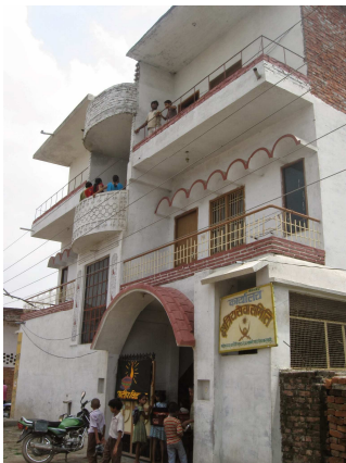
Here is the front of the building with some students standing in front of the main gate. We took them to see the new building for the first time yesterday.
