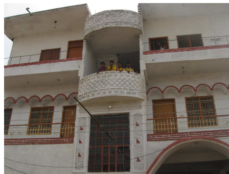
Here is a straight-on view of the front; the arch of the gate shows at the lower right. On the second and third floors there are two rows of classrooms going straight back with a wide corridor in the middle (corresponding to where the
